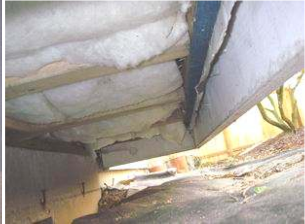
missing soffit
