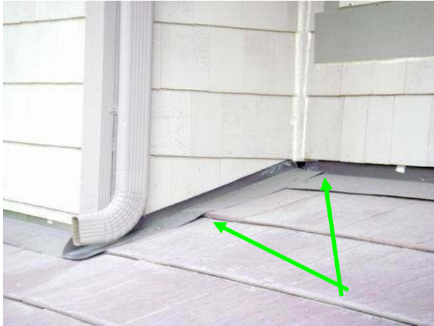
3 appear to be potential sources of moisture intrusion in a wind-driven rain
