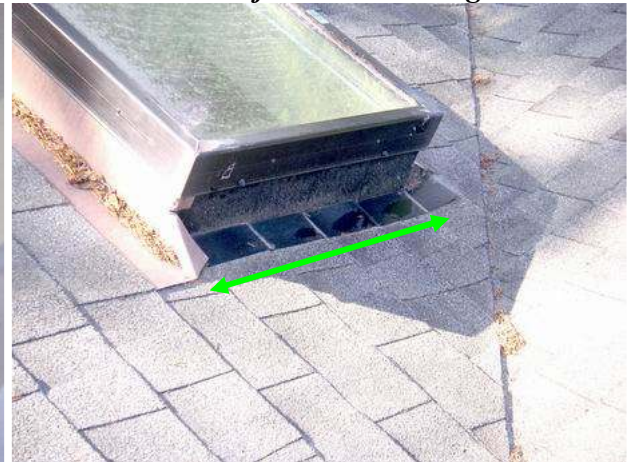
17 step flashing installed on top of shingles
