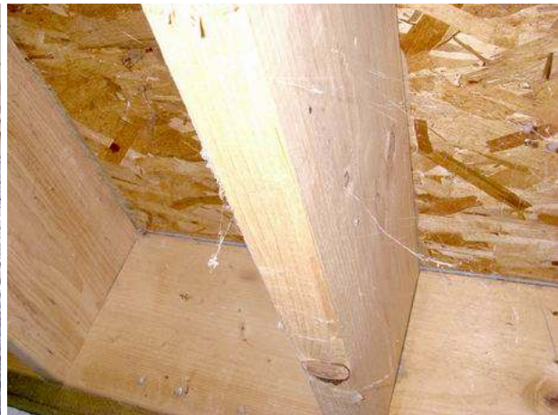
18 exposed framing underneath
