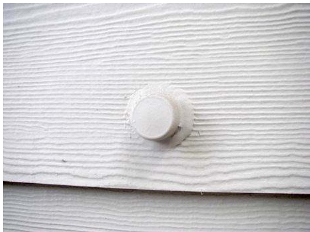
18 improper loop by-passes the air gap exterior air gap (should be drilled for air passage)
