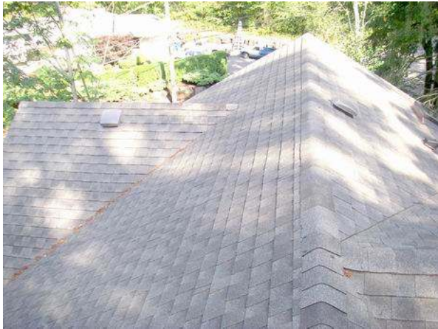
14 laminated architectural-style shingle roof
