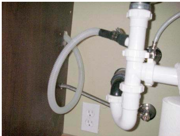
18 improper loop by-passes the air gap exterior air gap (should be drilled for air passage)
