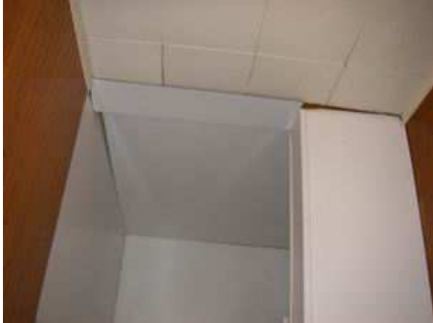
9 10 partial view of master bath ceiling
