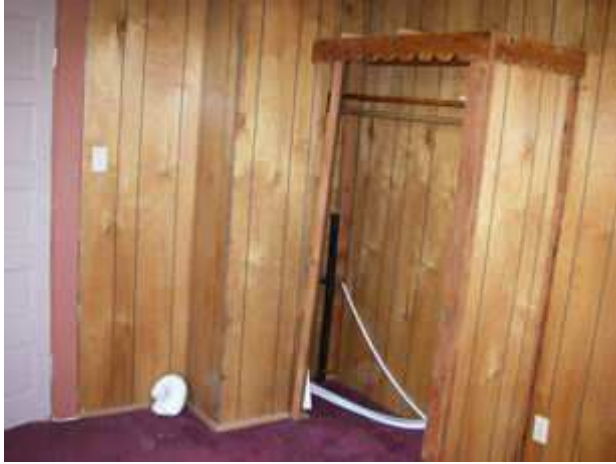
“closet” in master bedroom
