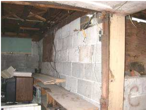
25 top three rows of block are rotating outward
