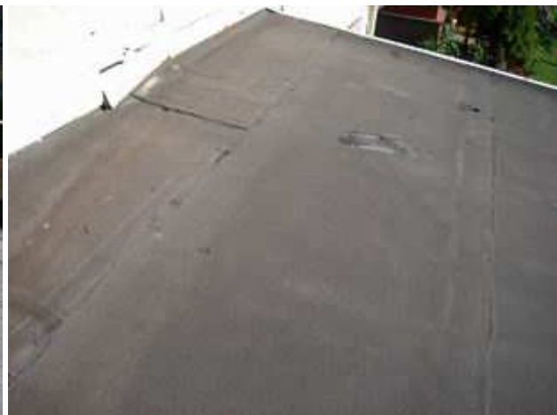
14 torchdown roof over front porch
