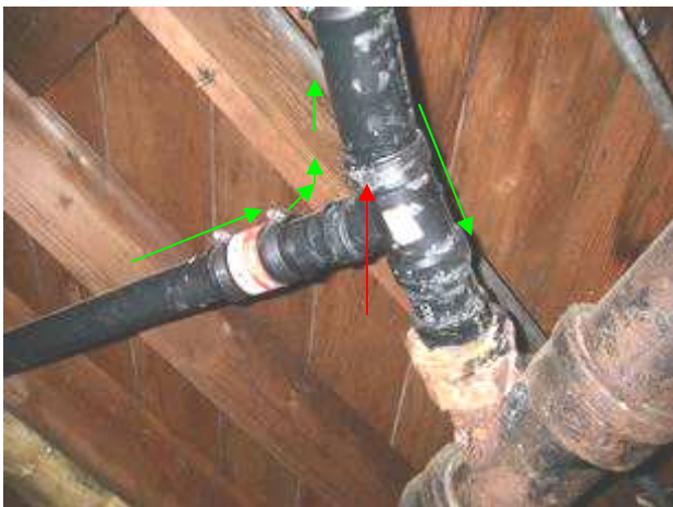
17 water must flow uphill prior to draining & one union attached at sharp angle\
