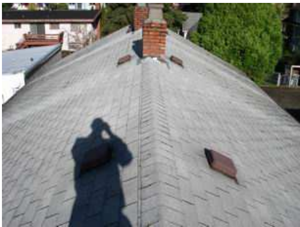
13 three-tab shingle roof
