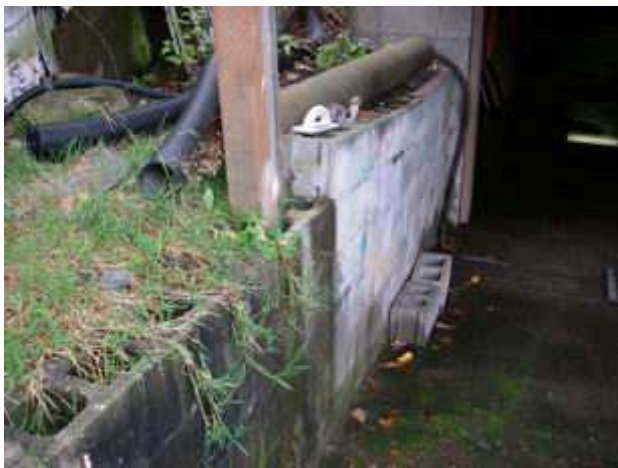
13 14 driveway retaining wall
