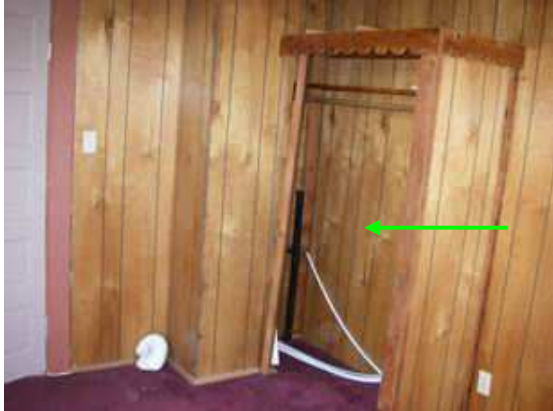
laundry vent capped in "closet"
