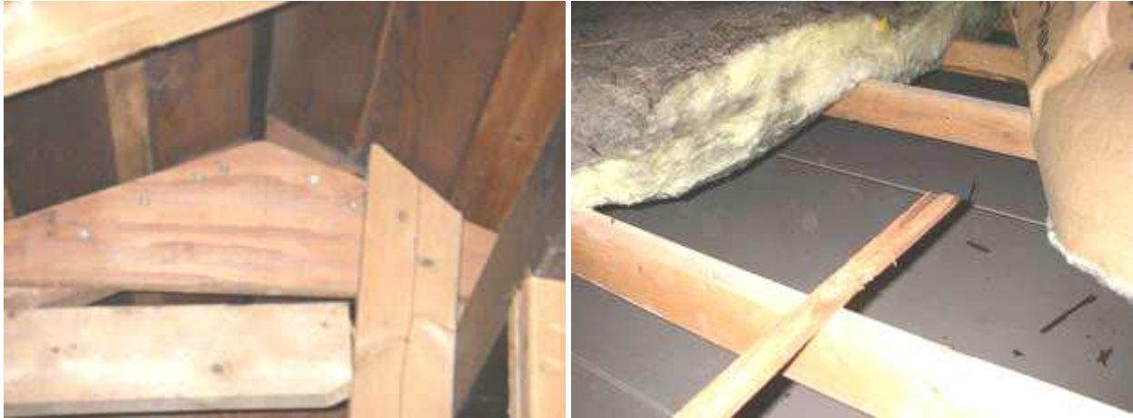
different views of retrofit roof framing & augmentation
