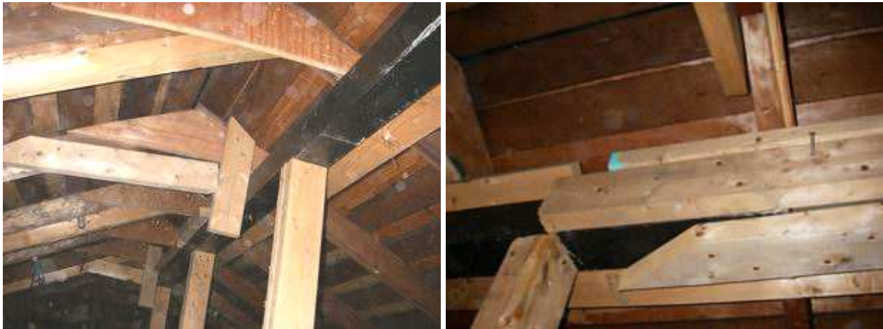
26 27 different views of retrofit roof framing & augmentation
