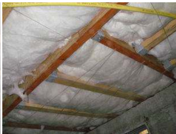
21 properly installed hangers at fireplace
