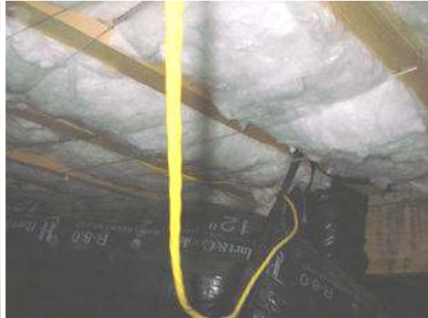
7 sagging conductor
