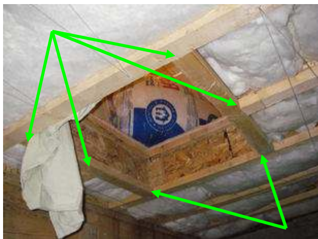
20 joist hangers & nailers required at these points
