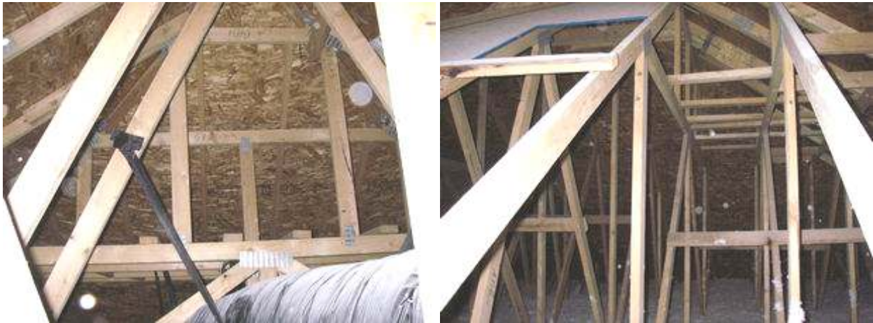
15 16 roof framing, typical
